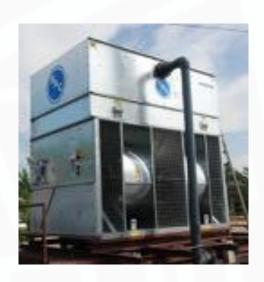
Counter flow, centrifugal fan, forced draft (single air intake)
