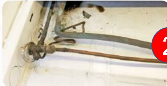
Removal of existing electronic controller and replacement of the mechanical thermostatic valve with an EEV.
