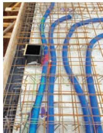
Figure 12: Scheme central ventilation units (top, middle), pipe laying in concrete (bottom) ©J. Pichler GmbH
