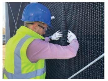
Figure 28: Heat transfer surface
