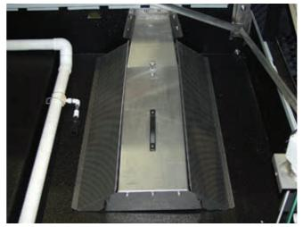
Figure 21: Cold water basin strainer
