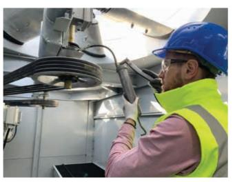
Figure 27: Greasing the bearing
