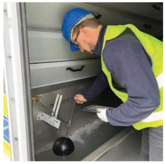
Figure 24: Mechanical water level control
