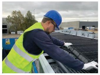
Figure 29: Drift eliminators
