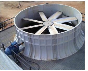
Figure 32: Mechanical drive system
