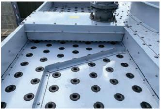
Figure 23: Hot water basin with gravity water distribution
