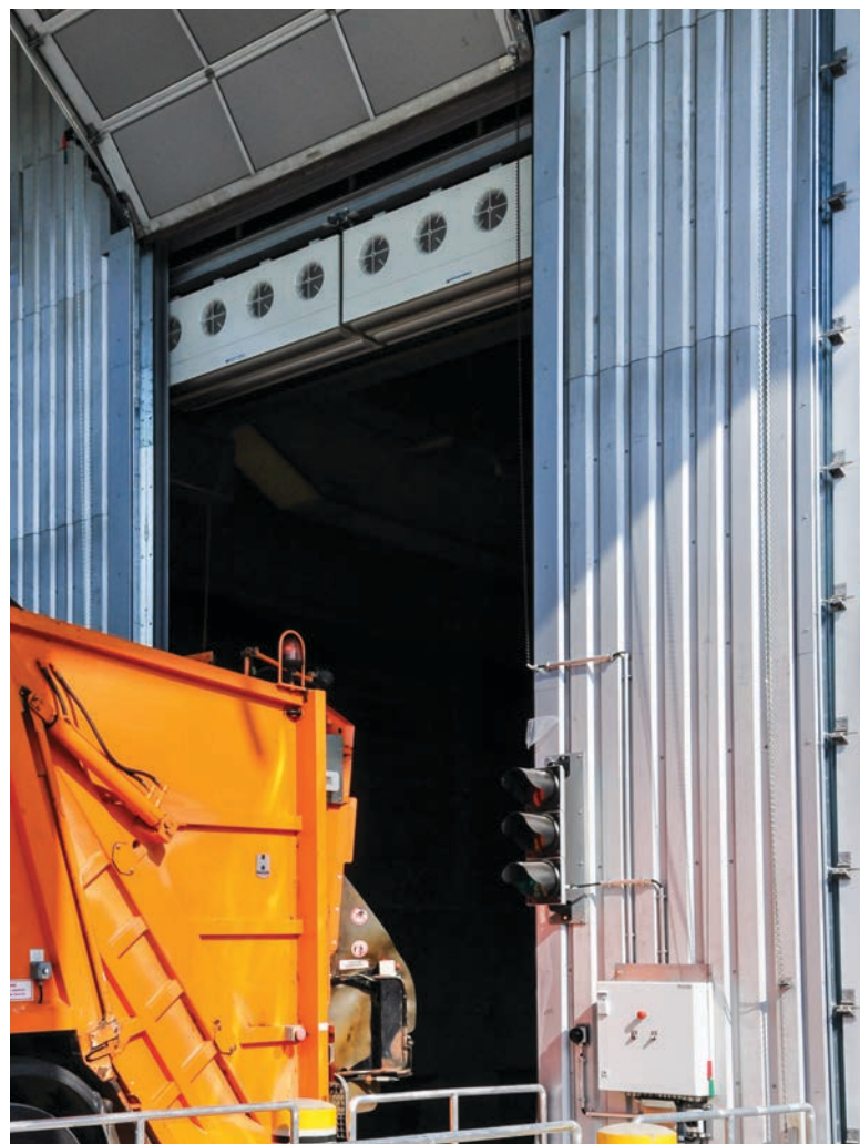
Figure 8 - Industrial Air Curtain
