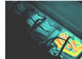
Uneven Heating in Trafo
