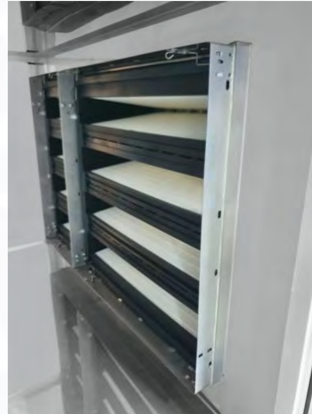
FILTER MOUNTING ARRANGEMENT
